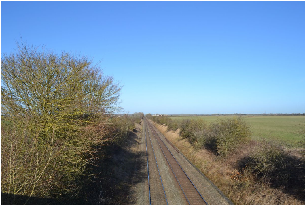
Photograph 131: View north-west along the railway line from the southern boundary of the former deer park.
