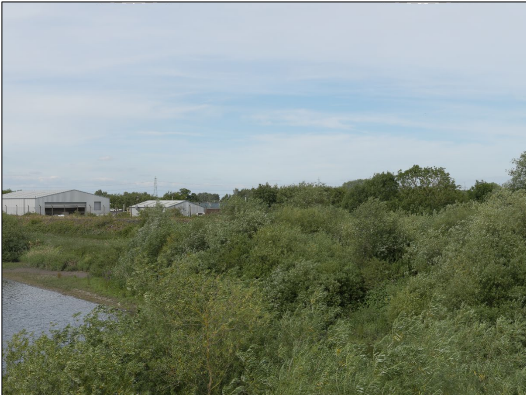
Photograph 42: View north-east Torksey Viaduct towards the West Burton 3 Site.
