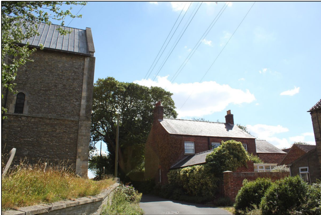
Photograph 19: View south illustrating the screening afforded by the built environment on the western side of the Site of a college and Benedictine Abbey, St Mary's Church, Stow (NHLE 1012976).
