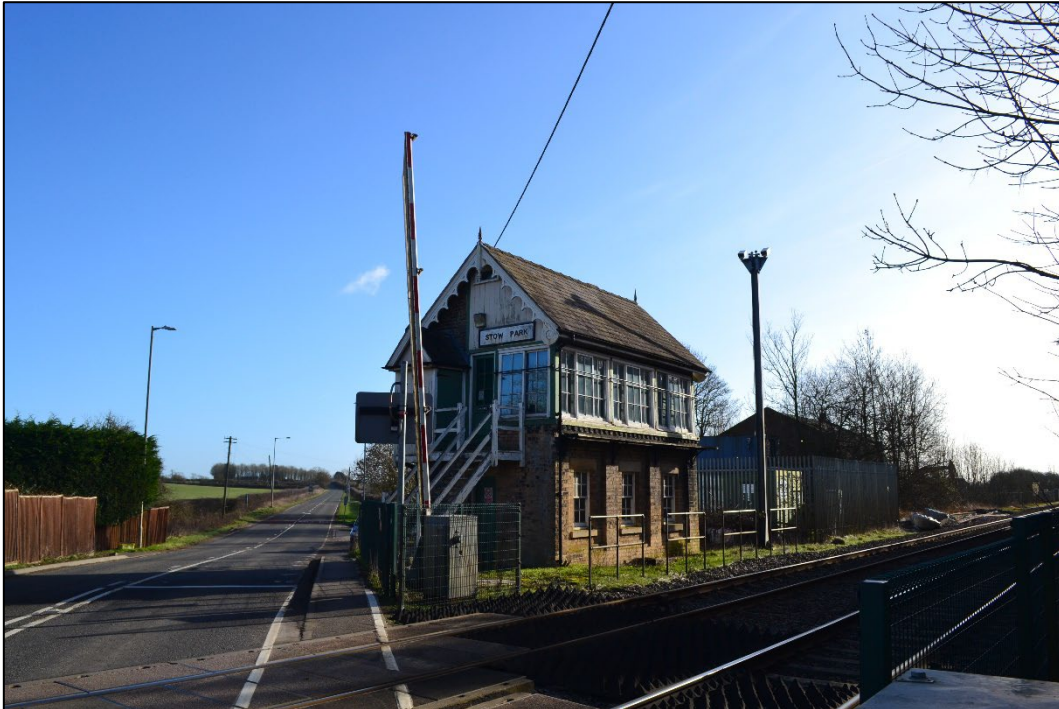
Photograph 73: View south-east from Till Bridge Lane towards the Signal Box at Stow Park Station (NHLE 1146606).
