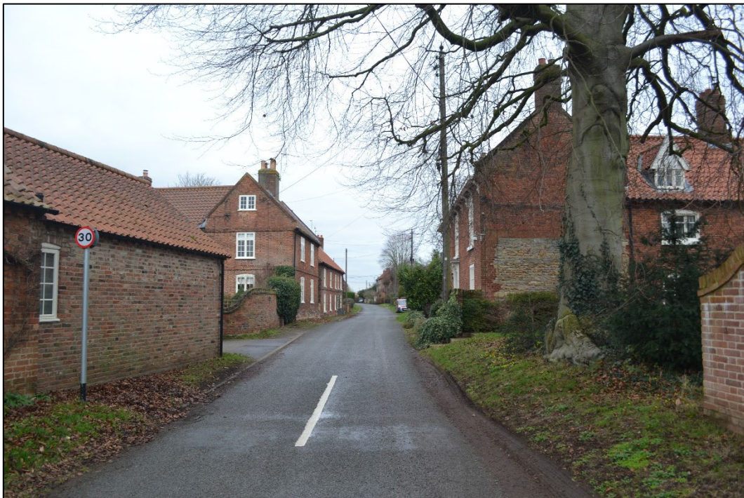
Photograph 52: View north along Brampton Lane from south of the Grade II Listed The Beeches, Richard-Havercross Cottages, and The Hermitage.
