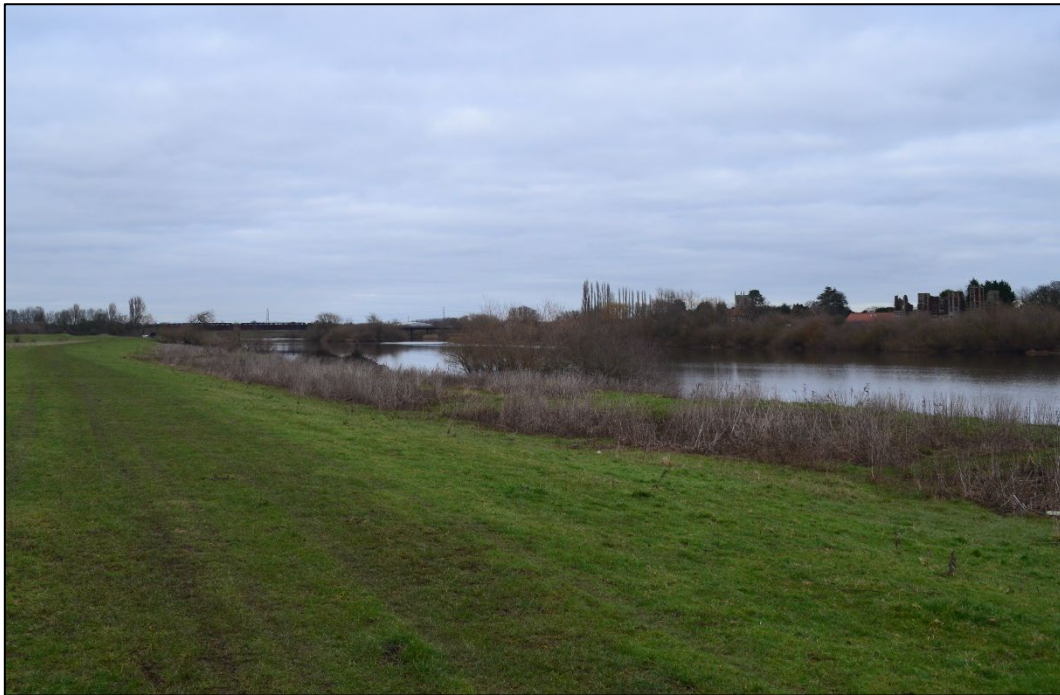
Photograph 43: View north towards Torksey Viaduct from the PRoW along the western bank of the river Trent.
