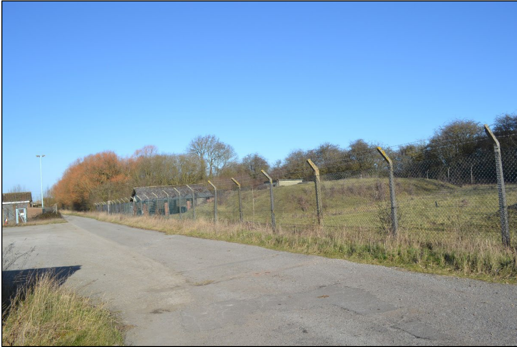
Photograph 128: View north-west from the access road adjacent to the MoD Petroleum Storage Depot.
