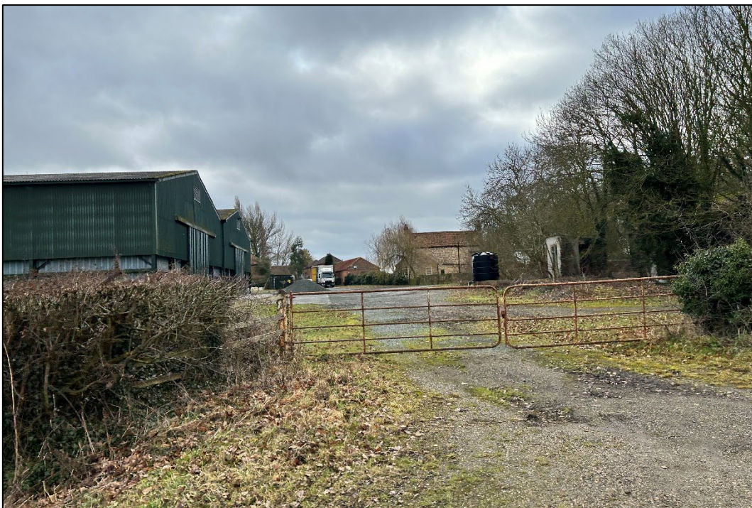
Photograph 60: View south from the Carlton Lane farm access towards the northern elevation of the Grade II Listed Cornhill Farmhouse (NHLE 1064096).
