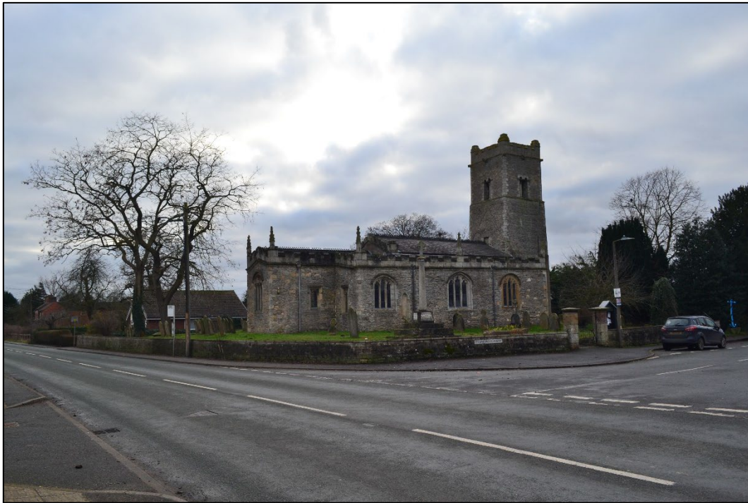
Photograph 65: View south-east of the Grade I Listed Church of St. Margaret of Antioch and the Grade II Listed Cross (NHLE 1146582) within the churchyard.
