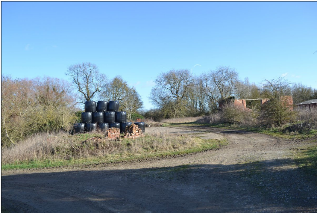
Photograph 125: View east across the central area of the site of the Bishop's Palace now occupied by hardstanding and derelict buildings associated with Moat Farm.
